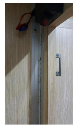
**Step 17**Connect the LED light strip to the Light box Switch
